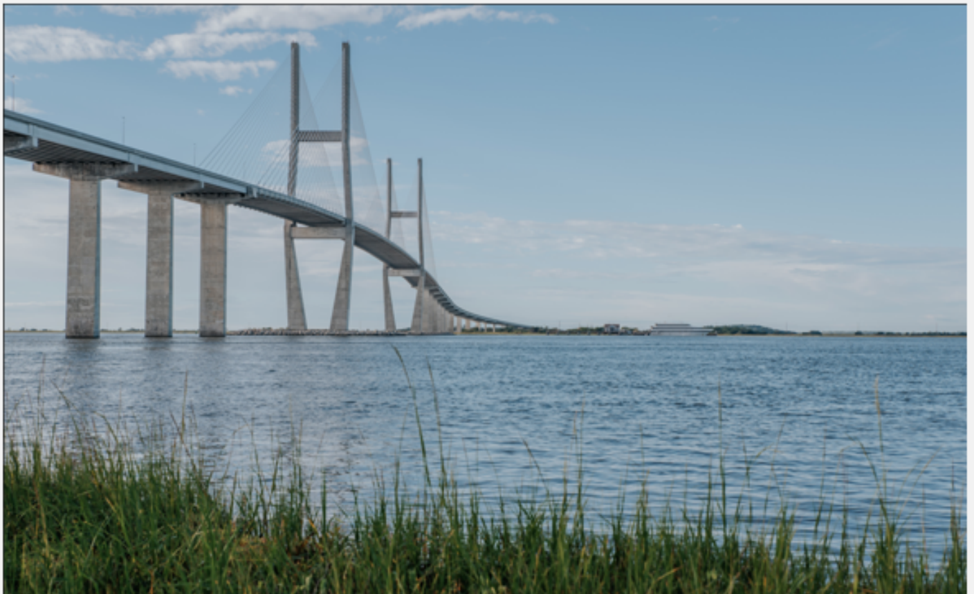
Sidney Lanier Bridge Brunswick, Georgia
